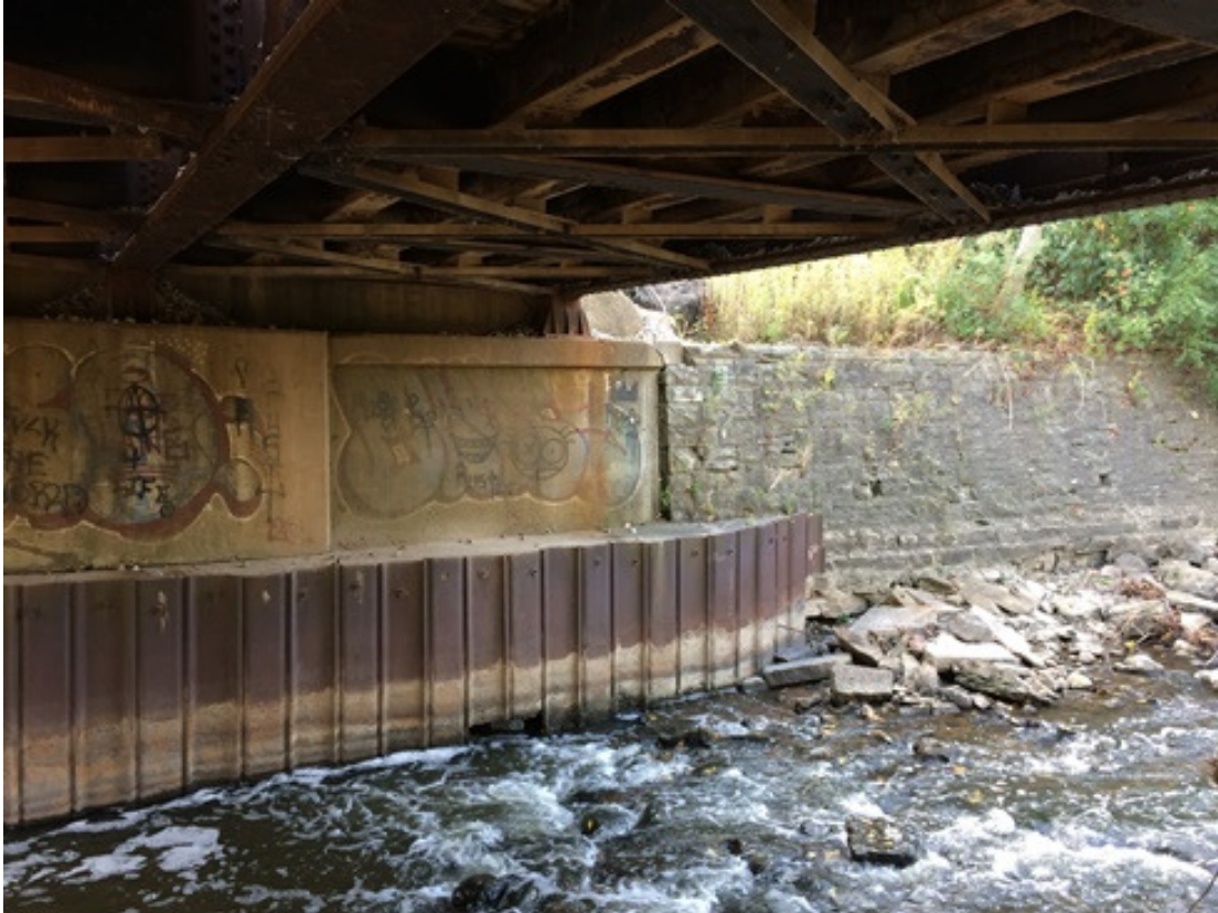
Photo 2 – Looking southeast at Abutment 1 of BR 88.74.
