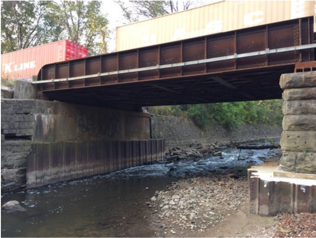
Photo 1 – Looking southeast at Abutment 1 of BR 88.74.
