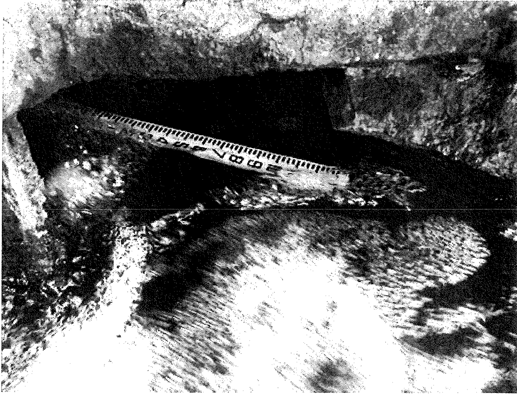
Photo 5 – Full extension of 13' long tape measure under the Abutment 1 footing.
