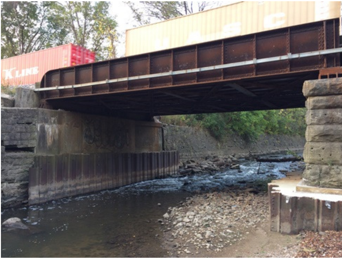
Photo 1 – Looking southeast at Abutment 1 of BR 88.74.
